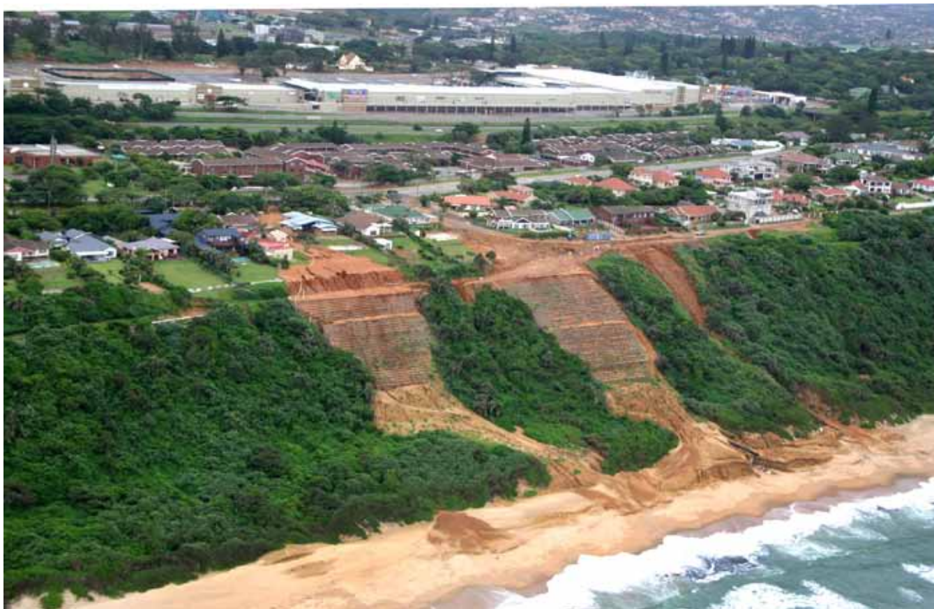
Durban's coastline is vulnerable to erosion. © eThekweni Municipality
